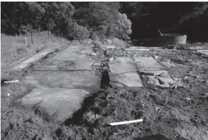
6 (top). The collapsed outbuilding immediately prior to investigation.
