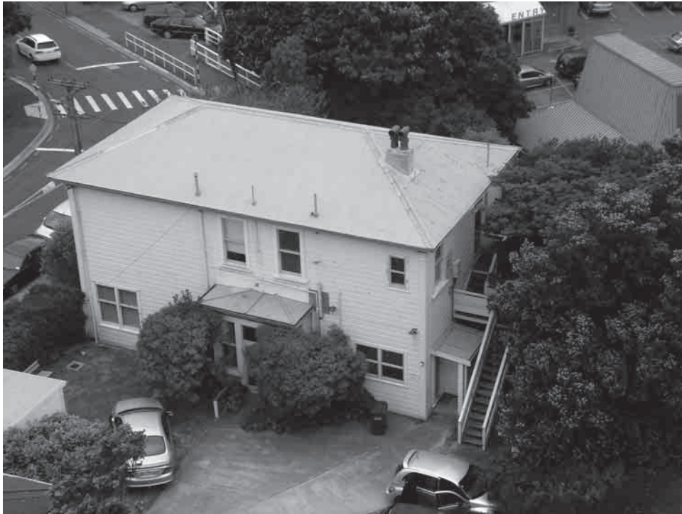
4.8. 5 Pipitea St from south west, above. The staircase and covered entrance on the right are the later additions (photo: Arcad).
