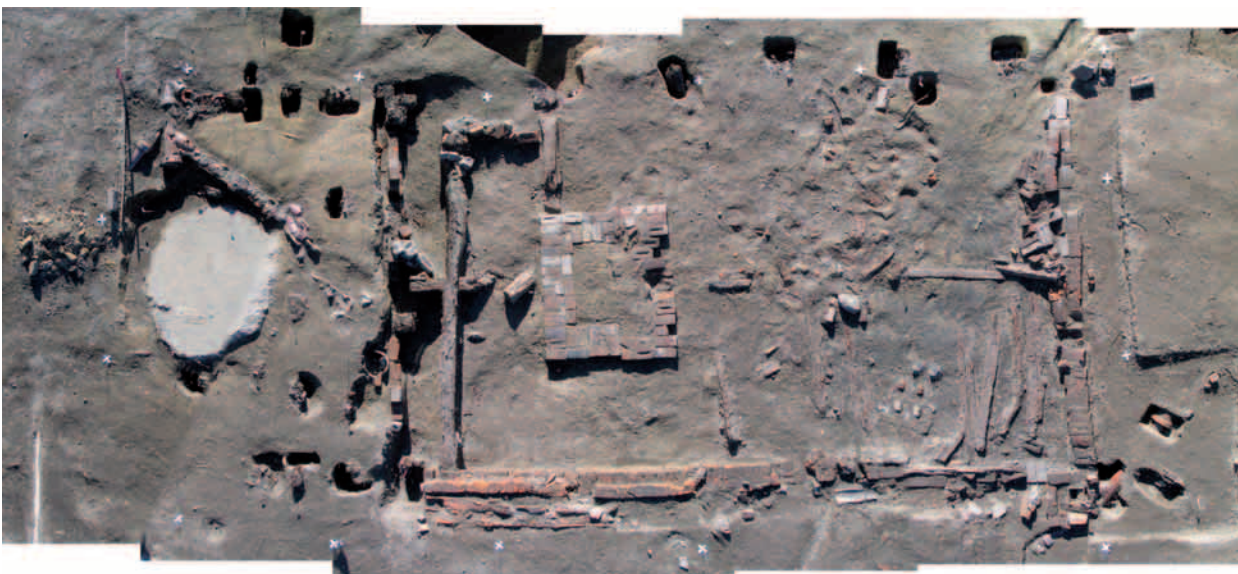
5.8. Topdown composite photo of the Phase 3 extension to the back of 3 Pipitea Street, showing the collapsed subfloor framing.
