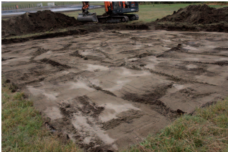
5. Trench 3 after excavation.
