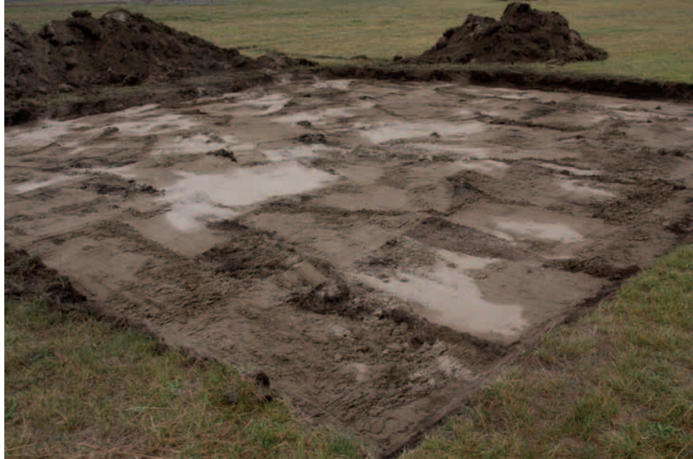
4. Trench 2 after excavation.
