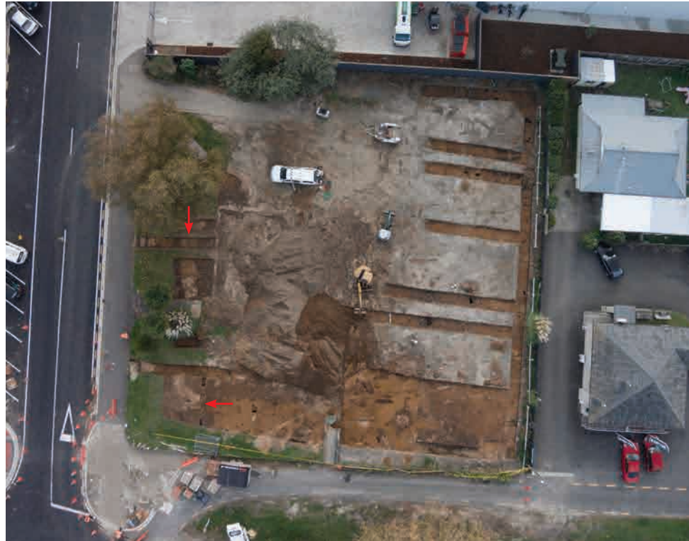
8. Aerial photograph showing the path curving around the corner of the old building (arrowed). It appears to be truncated at the point where building phases 8 and 9 created the lean-to.
