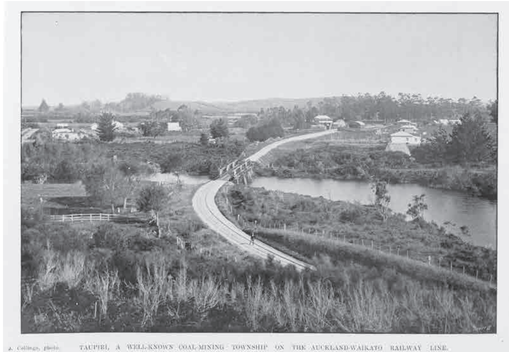
2. View of the original bridge alignment taken in 1906 looking south toward Taupiri. (NZG_19060818_7_2, photographer J. Collings, Sir George Grey Special Collections, Auckland Libraries)
