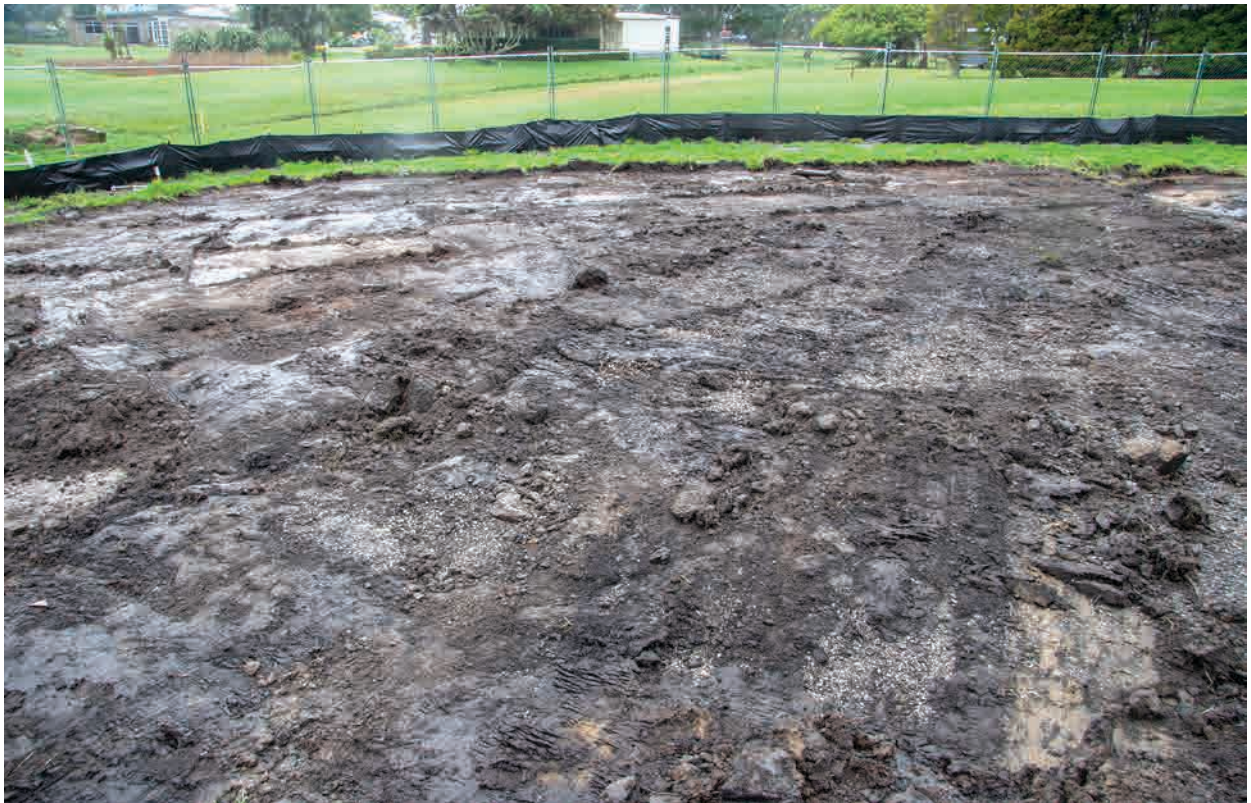
Figure 9. (9727) T12/221 exposed after topsoil stripping for fill.
