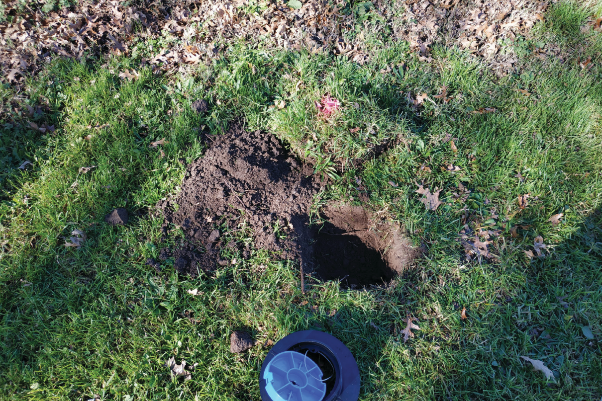
Figure 9. Typical pit dug for installation.
