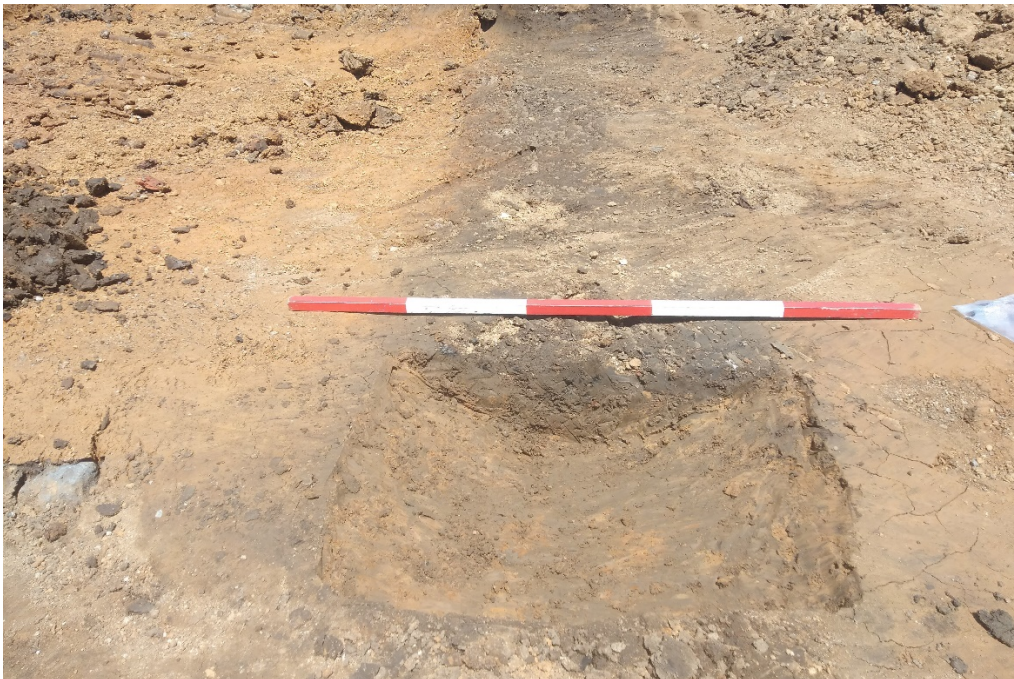
Figure 9. Cut and fill within drain feature for farm buildings that extended east to west across the building platform for Units 7-22 then turned north towards the new driveway
