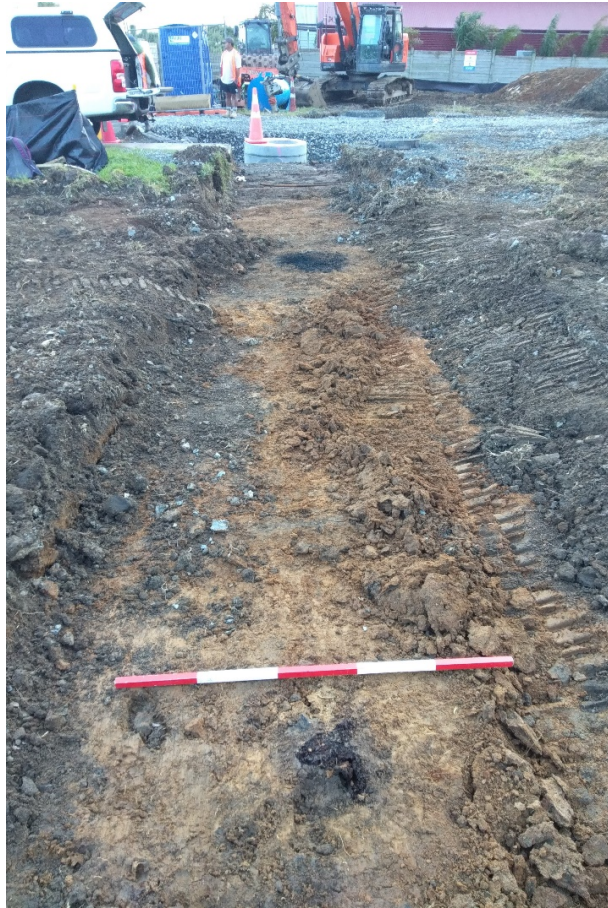
Figure 4. Area stripped to clay for wastewater drain for Units 7-22, showing post-holes below demolition layer.
